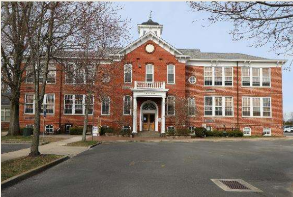
Old Cranbury School, 23 North Main Street
